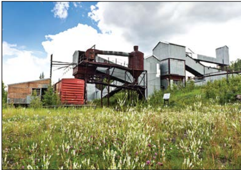
The Brazeau Collieries Briquette Plant
